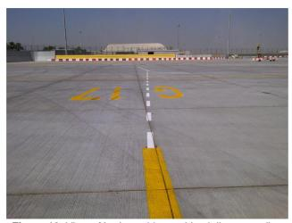
**Figure 10.** View of broken white pushback line extending from the G17 stand centerline to a T-stop mark. The jetblast fence is on the left hand side of the stand in this view
