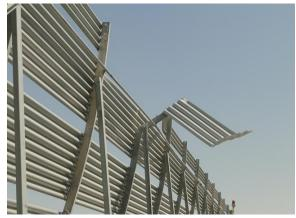
Figure 6. Damage to blast fence
