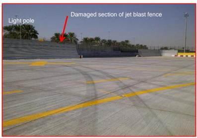
Figure 13. A6-ENK main gear tire marks
