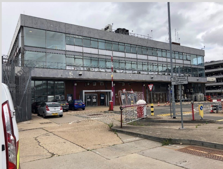
Figure 6: D'Albiac House, Heathrow Central Terminal Area
